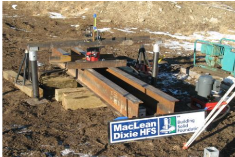
Full scale field testing- compression/tension/lateral
