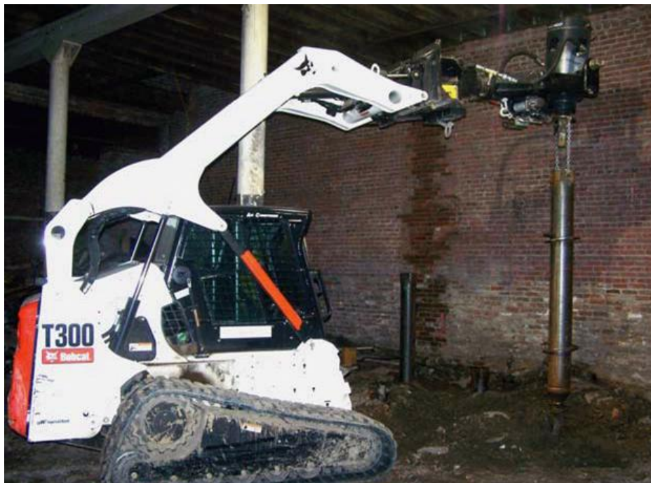
Foundation Repair with P8 in Limited Access Location (9-story structure)
